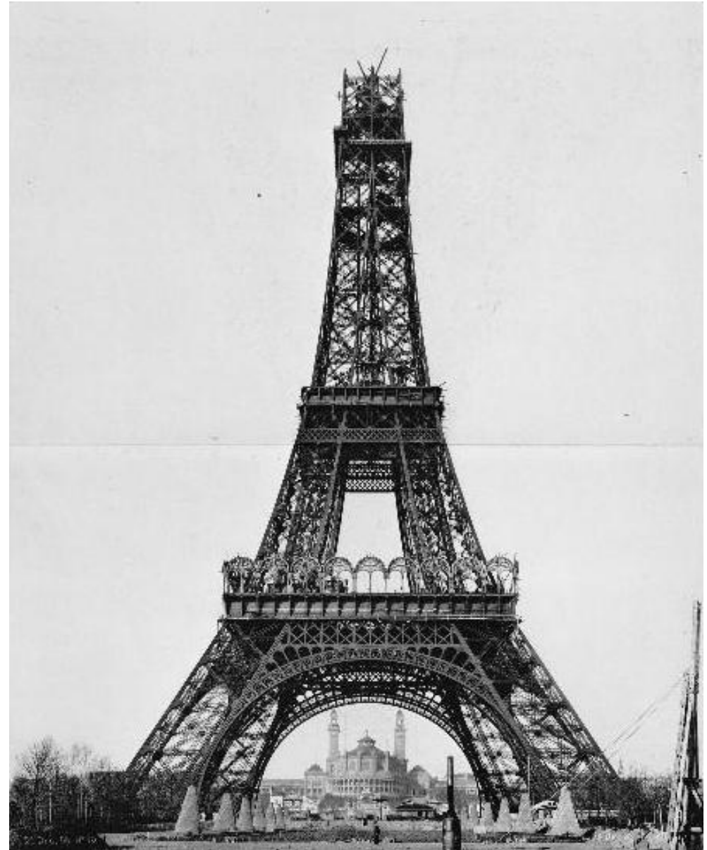
Construction of the Eiffel Tower, December 1888
