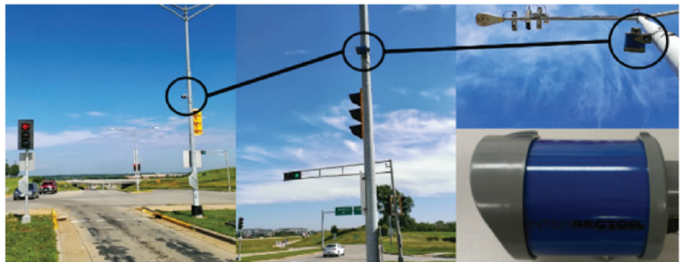
Typical Installation of Radar-Based Vehicle Detection System on Signalized Intersection
