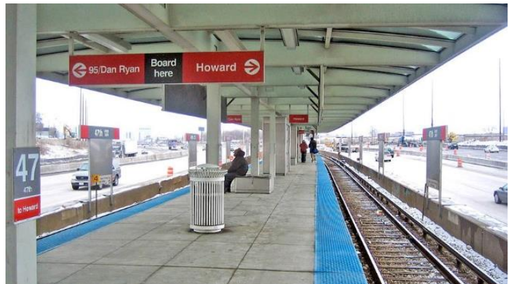
Figure 11. The Chicago Transit Authority's Red Line is one of several U.S. mass transit facilities located in freeway medians. An electrified third-rail is visible at the lower right. Photo: Graham Garfield/WikiMedia Commons
