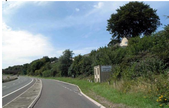
Figure 14. Emergency Parking pull-out with storage shed for emergency traffic control devices (permanent site).
