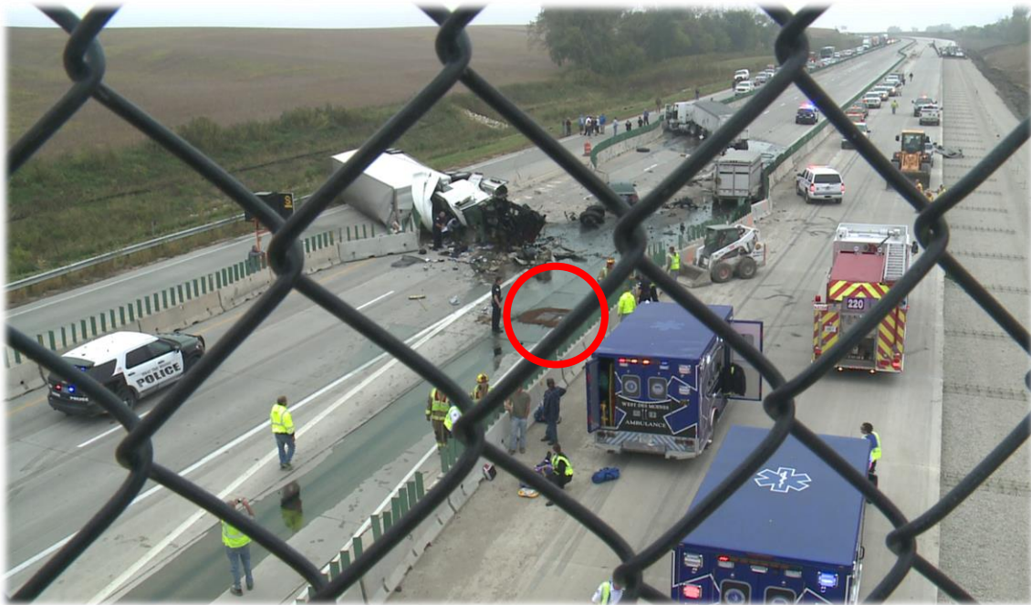
Figure 23. I-35 crash site near West Des Moines, Iowa, viewed through the fence from an overpass. The concrete barrier was heavily damaged. Responders used the lanes that were closed for construction to reach the site. This view also illustrates contractor personnel and equipment placing soil to block spilled diesel fuel from entering the storm drain (red circle). Photo: West Des Moines Police Department
