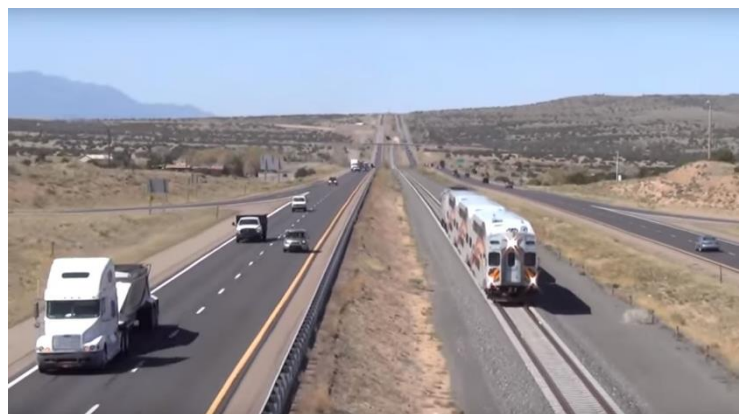
Figure 12. New Mexico Rail Runner, a commuter train connecting Belen, Albuquerque and Santa Fe, operates partly in the median of I-25. Photo: Aaron Friedman/YouTube
