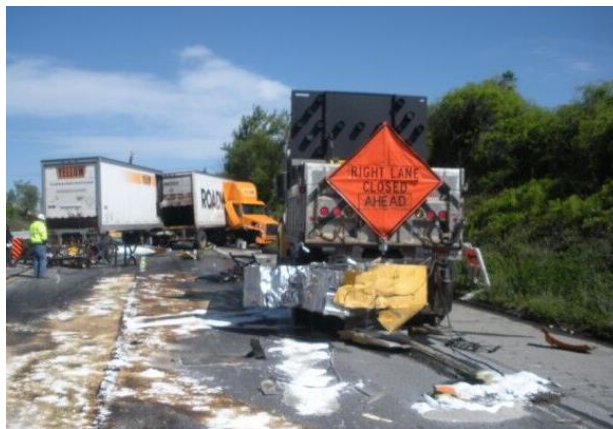
Figure 19. Spreading absorbent material to soak up spilled diesel fuel. Photo: Pennsylvania DOT
