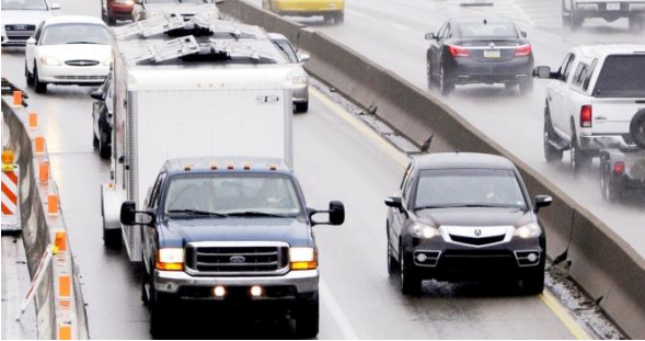
Figure 3. Work zones with barrier on both sides can be difficult to access in the event of an incident.
