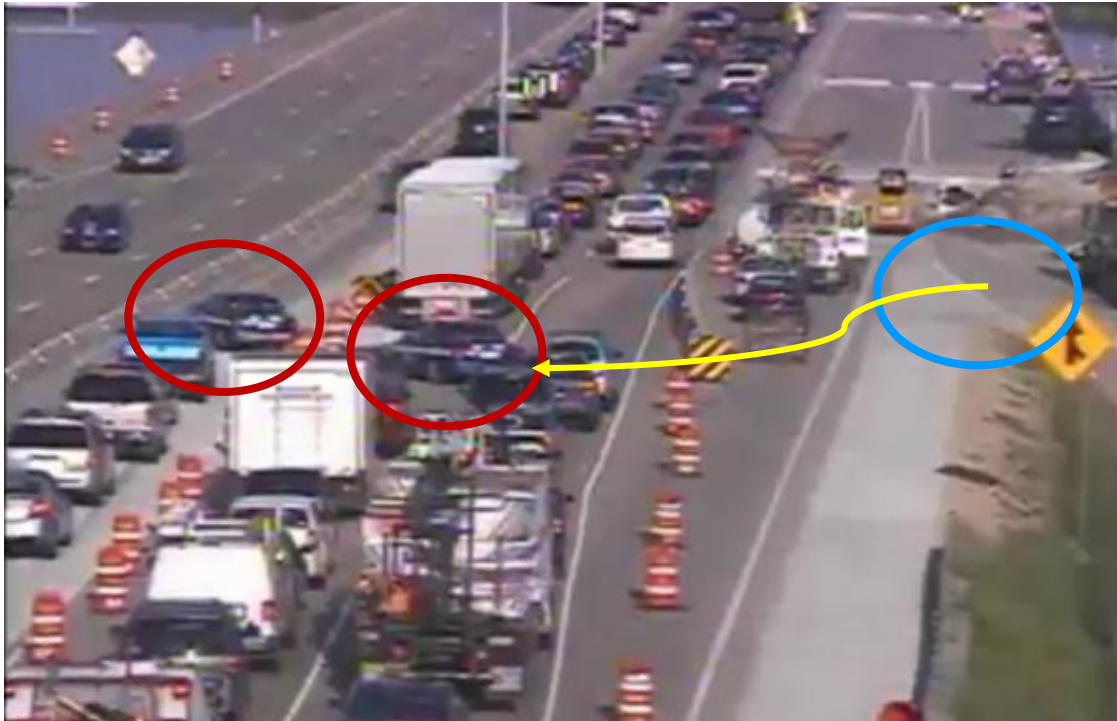
Figure 22. During the Madison (WI) Beltline work zone crash responders took advantage of the split lane configuration. Originally both police vehicles were staged at the closed entrance ramp identified by the blue oval. One responder used each side to assure that at least one squad would reach the incident site in a timely manner (red ovals). Photo: Wisconsin DOT
