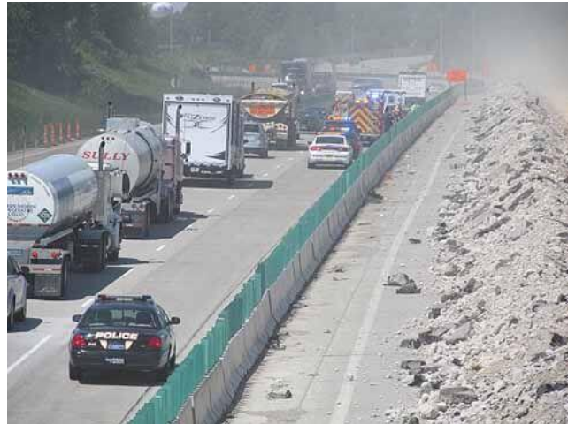
Figure 1. Traffic bottleneck from a work zone incident.
