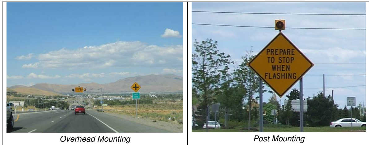
FIGURE 7.2 ADVANCE WARNING FLASHER MOUNTING OPTIONS
