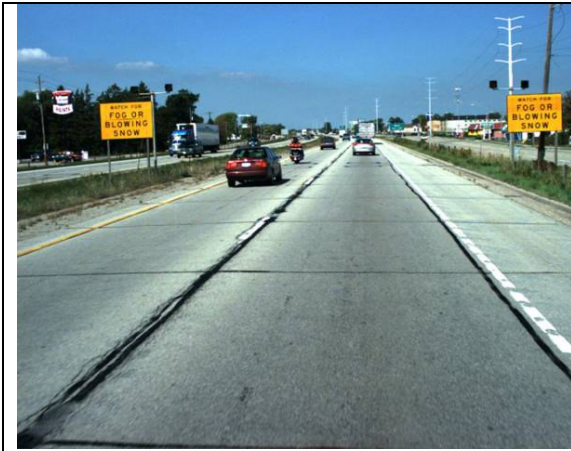
USH 41 northbound fog signs
