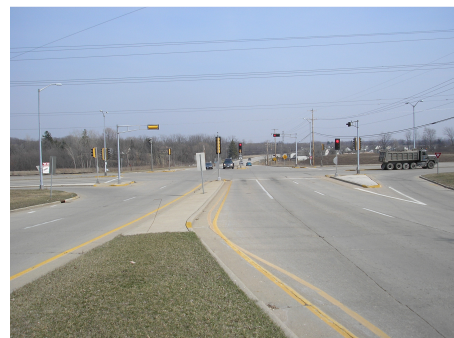
Example of a right-turn channelization island with the proposed configuration STH 59/164 and CTH D in Waukesha County
