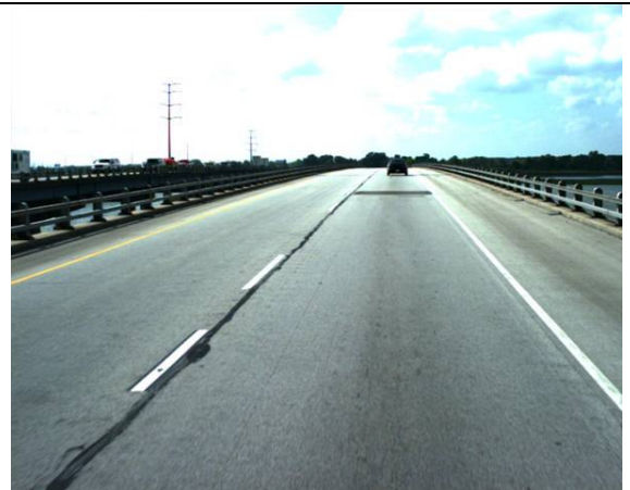
USH 41 southbound Lake Butte des Morts Bridge
