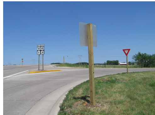
Right Turn Channelization Island on STH 26 and USH 41 Northbound On-Ramp
