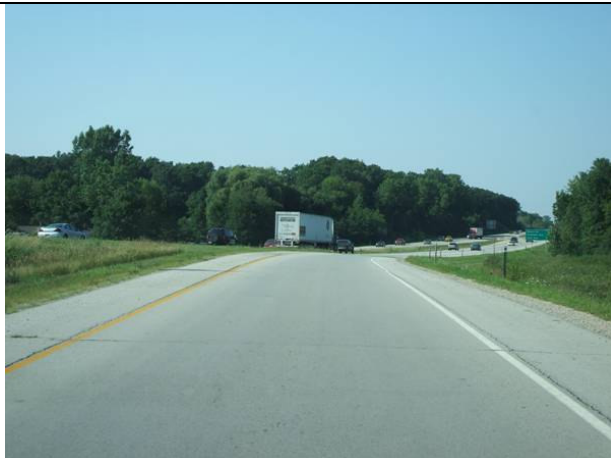
Lombardi Northbound On-ramp
