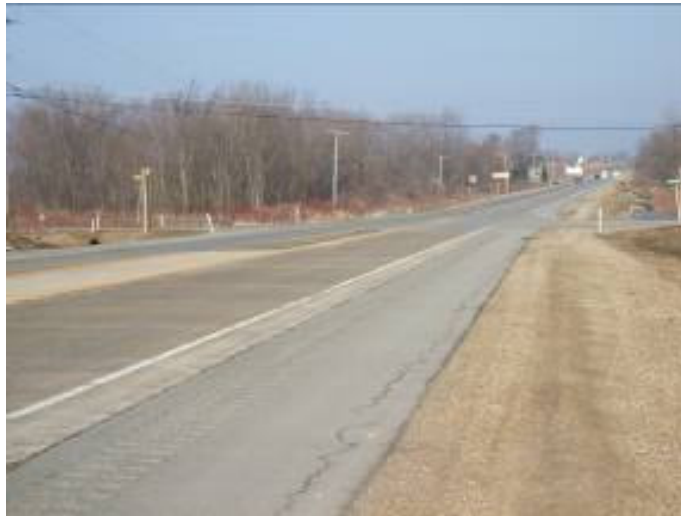
Rumble strips terminate to the east of Rock River Road intersection
