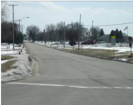
STH 16 and North Road intersection
