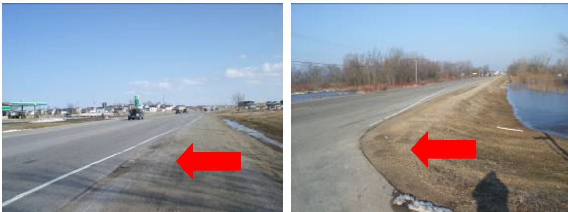
Paved shoulders not carried through taper sections at the intersections
