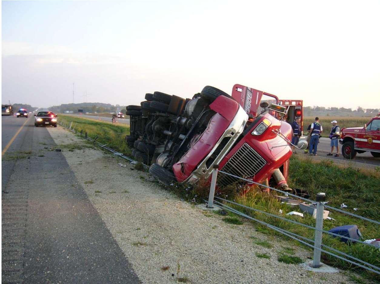
Figure 5 A Semi-Truck Stopped by Cable Barriers (Brifen).
