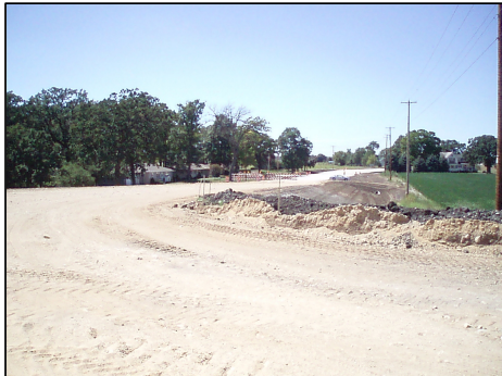
intersection of Bypass ramp with existing roadway
