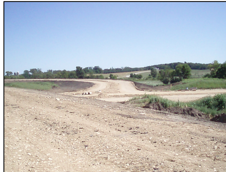
Bypass roadway (foreground) with jug-handle ramp (background)
