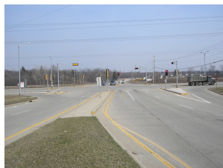
Example of a right-turn channelization island with the proposed configuration (STH 59/164) and Cleveland in Waukesha County
